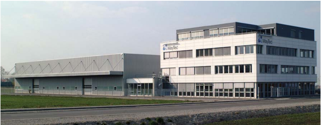
MayTec GmbH plant in Dachau
